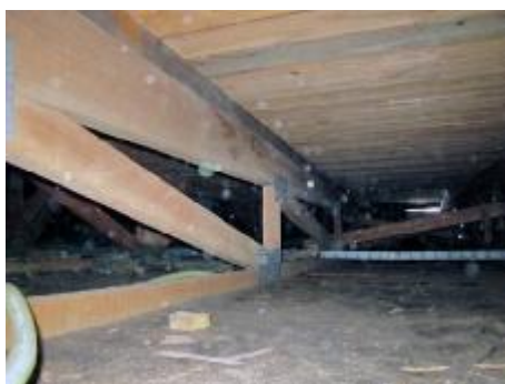
Figures 27 and 28. Flat roof (left). Batten nails not fixed in roof trusses (right)
