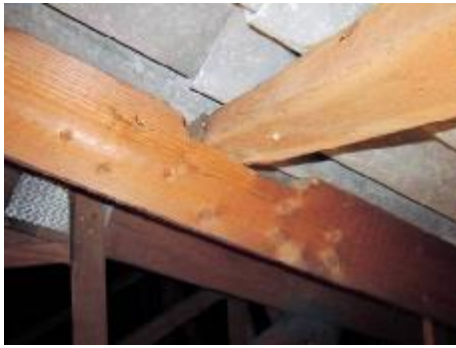
Figures 29 and 30. Reduced cross section of trusses (left). Attic used as a warehouse (right)
