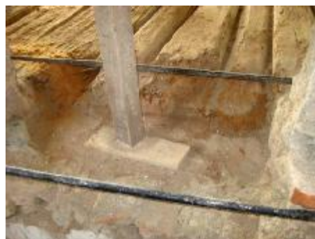
Figures 9 and 10. Complete deterioration of hollow timber floor (left). Massive timber floor – damage caused by brown rot (right)
