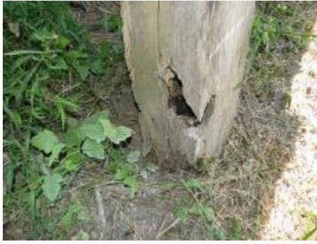
Figures 39 and 40. Reduced cross section of pillars
