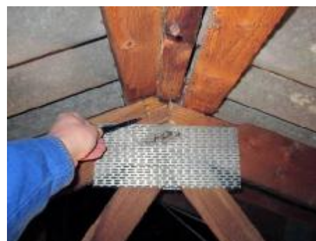
Figures 27 and 28. Flat roof (left). Batten nails not fixed in roof trusses (right)
