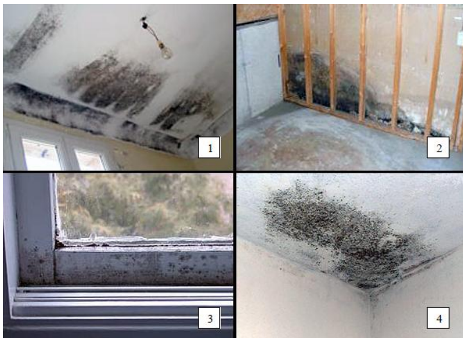
c) Vлага uzrokovana termičkim mostovima je dobra podloga za nastanak plesni [22] c) Moisture induced by thermal bridges is a good substrate for the development of mould [22]
