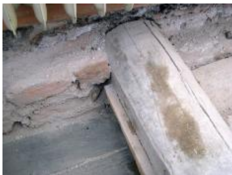
Figures 21 and 22. Hollow timber floor joist (left). Deterioration of joists (right)
