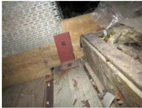
Figures 31 and 32. Fixation of trusses to frame walls (left). Fixation of trusses to concrete walls (right)
