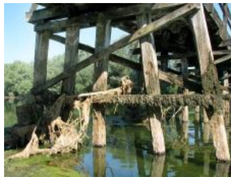
Figures 37 and 38. Dilatation profile not installed (left). River debris (right)
