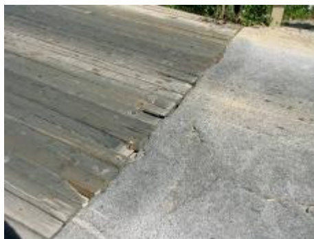
Figures 37 and 38. Dilatation profile not installed (left). River debris (right)
