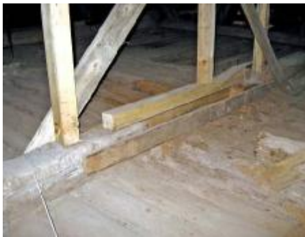
Figures 5 and 6. The lower chord of the main girder was completely deteriorated (left). Several ad-hoc renovations were made (right)
