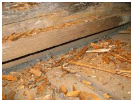
Figures 21 and 22. Hollow timber floor joist (left). Deterioration of joists (right)
