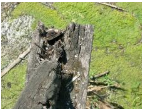
Figures 41 and 42. Deteriorated pile bracing (left). Deterioration of longitudinal chords (right)
