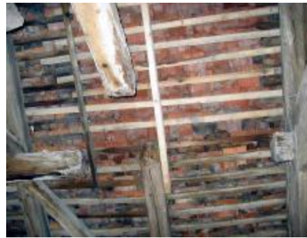
Figures 5 and 6. The lower chord of the main girder was completely deteriorated (left). Several ad-hoc renovations were made (right)
