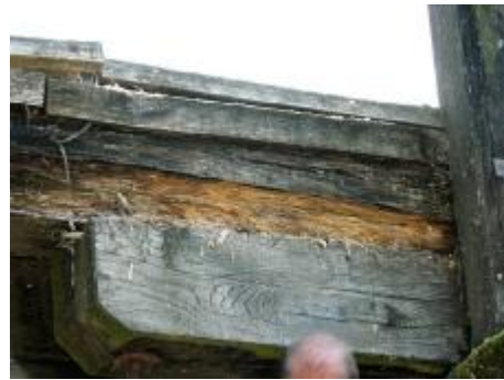
Figures 41 and 42. Deteriorated pile bracing (left). Deterioration of longitudinal chords (right)
