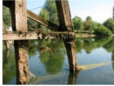
Figures 39 and 40. Reduced cross section of pillars
