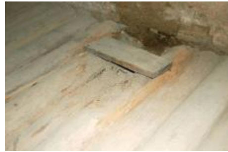
Figures 17 and 18. Damage caused by house capricion (left). Damage primarily caused by fungi - brown rot (right)
