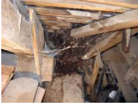
Figures 3 and 4. Timber deterioration in the gutter valley
