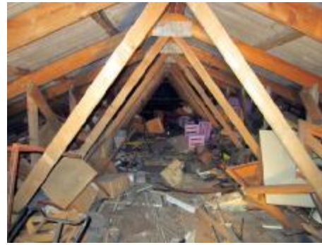
Figures 29 and 30. Reduced cross section of trusses (left). Attic used as a warehouse (right)
