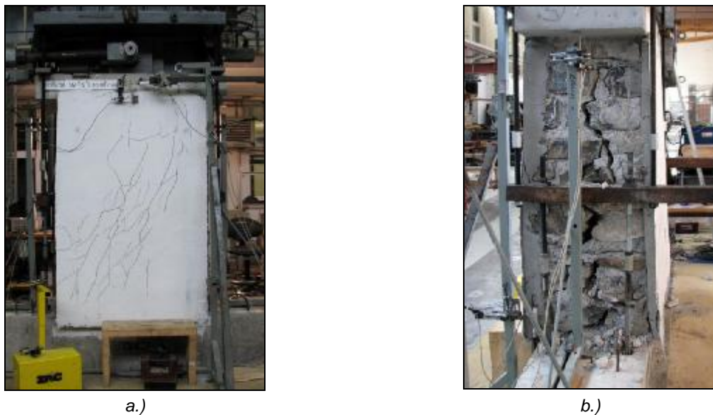
Figure 8. Stone masonry, strengthening type 2: a.) cracks in the coating at ultimate state; b.) separation of the wall's wythes
