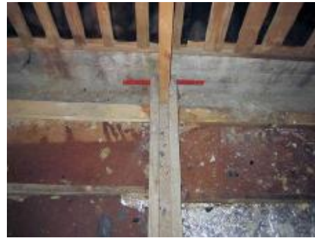
Figures 31 and 32. Fixation of trusses to frame walls (left). Fixation of trusses to concrete walls (right)
