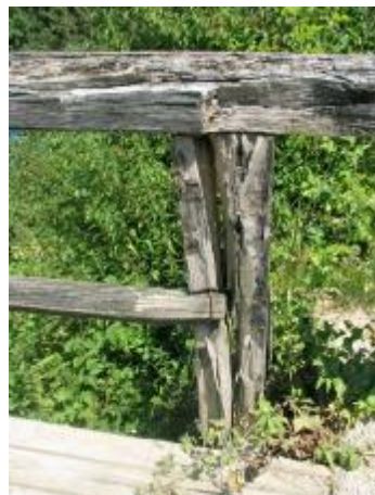
Figures 43 and 44. Deterioration pile caps (left). Deteriorated railing (right)
