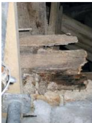
Figures 9 and 10. Complete deterioration of hollow timber floor (left). Massive timber floor – damage caused by brown rot (right)
