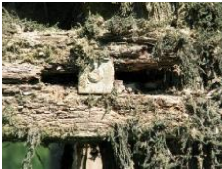
Figures 41 and 42. Deteriorated pile bracing (left). Deterioration of longitudinal chords (right)
