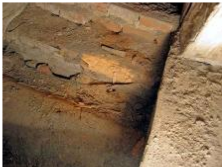
Figures 7 and 8. Damage due to insect attack (left). Clear identification of elements that should be replaced (right)
