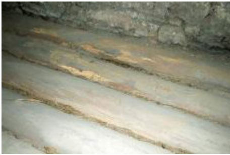
Figures 17 and 18. Damage caused by house capricion (left). Damage primarily caused by fungi - brown rot (right)
