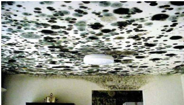
a) Razmnožavanje plesni u velikoj razmeri po plafonu na mestu spoja balkona sa tavanicom [4] a) A large-scale reproduction of mould on the ceiling at the location where the balcony meets the ceiling [4]
