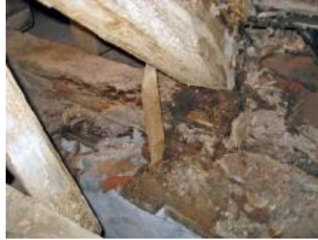
Figures 3 and 4. Timber deterioration in the gutter valley
