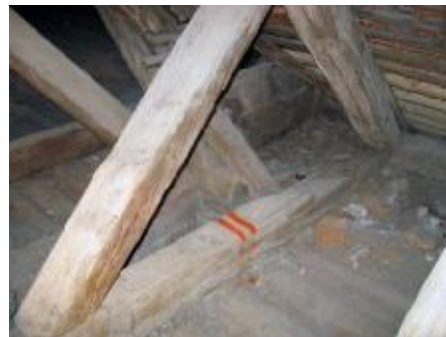
Figures 7 and 8. Damage due to insect attack (left). Clear identification of elements that should be replaced (right)
