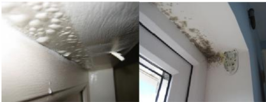
b) Kondenzacija se javlja na mestima bez izolacije i vremenom, bez dodatne ventilisanosti, pojavljuje se plesan [5] b) Condensation occurs in locations with no insulation; over time, without additional ventilation, mould appears in these locations [5]
