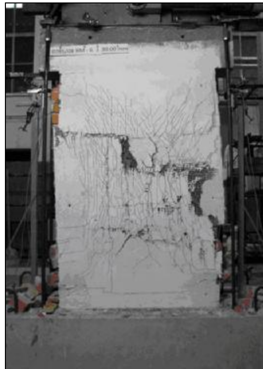
Figure 13. Brick masonry: strengthening type 14. Rupture of GFRP grid at ultimate state
